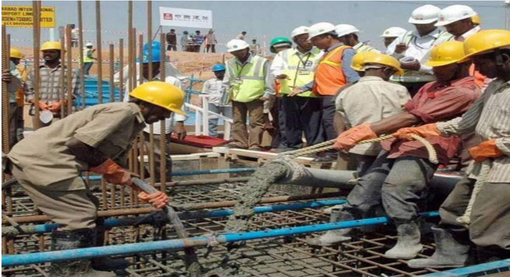
Fig.3: Placing and compacting concrete
